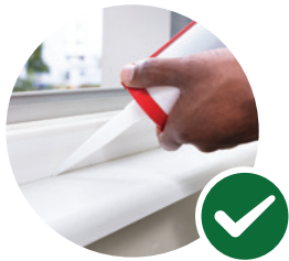
Seal gaps and cracks in doors and windows
